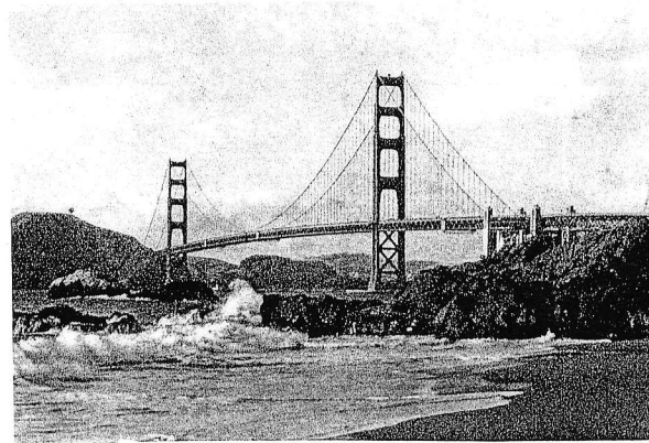
Golden Gate Bridge – California
